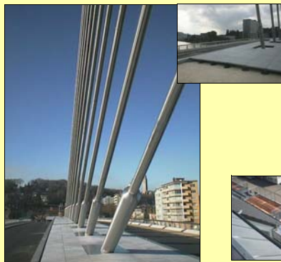
Val Benoit Bridge - Liège - Belgium
